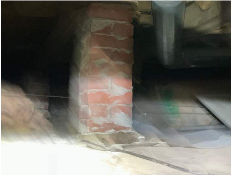
Masonry pier bearing on stone No frost protection
