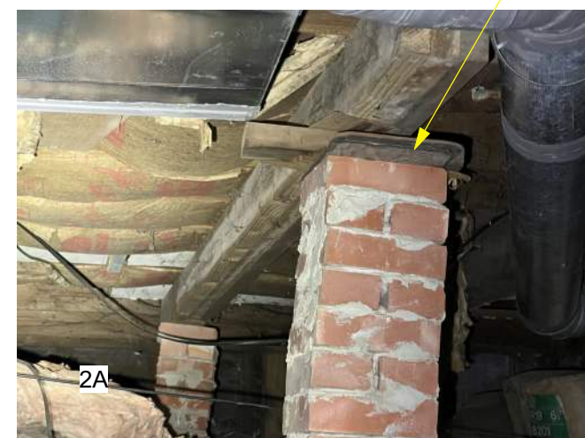
NOTICE POOR PIER CONSTRUCTION QUALITY
