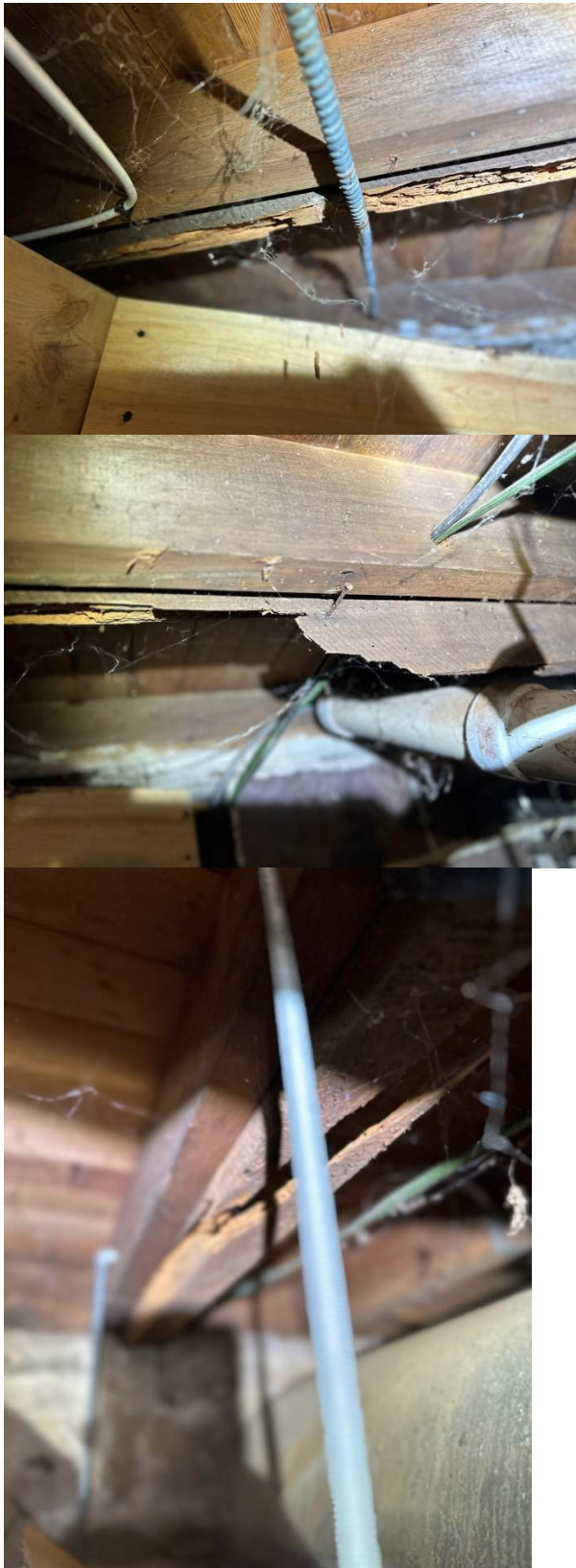
Deteriorated joist sistered
