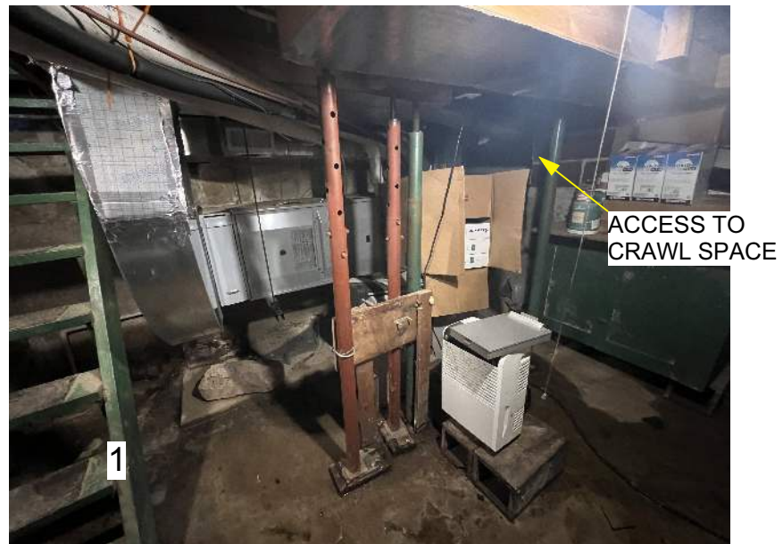
BASEMENT - NOTICE TEMP SUPPORT POSTS AND EXTREMELY CRAMPED CONDITIONS
