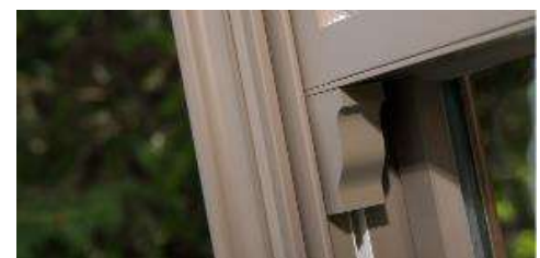
Flush Sash Lugs that Allow Tilting
