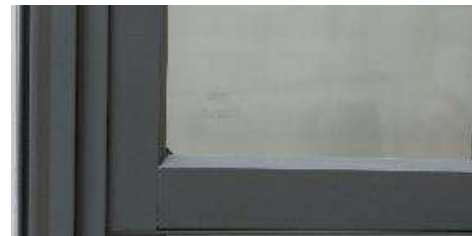
Through-Stile Construction
