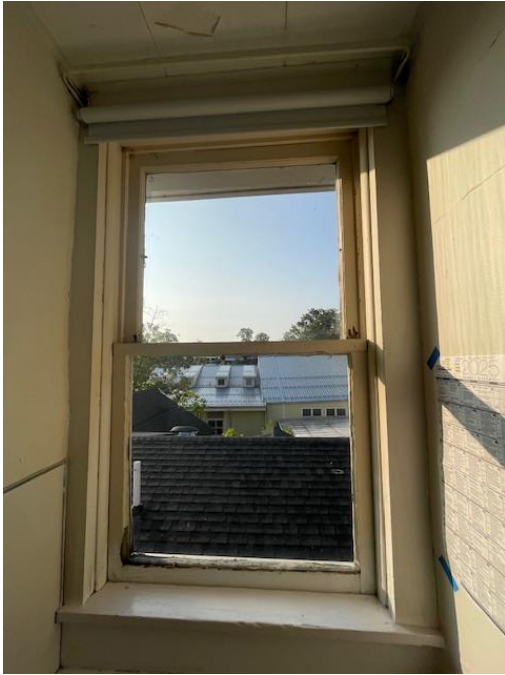
BW 25 - South – Rotted wood Missing operational hardware
