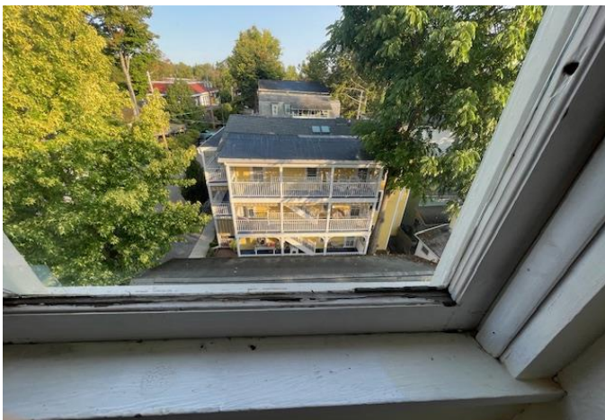
BW 26 North - No operational hardware Cracked glass Rotted wood
