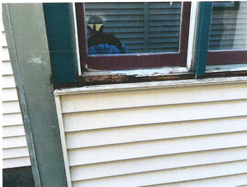
Typical window condition showing deteriorated sills and interior wall damage that was addressed last fall with a certificate of appropriateness. Window sash was filled with bond and painted to prevent additional wall damage till windows could be replaced.
