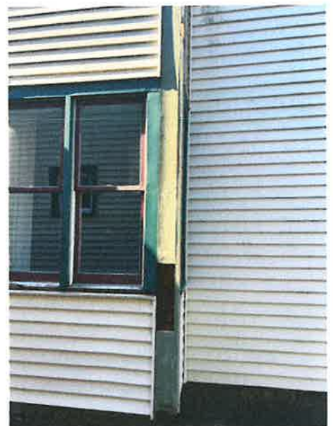
Typical window condition showing deteriorated sills and interior wall damage that was addressed last fall with a certificate of appropriateness. Window sash was filled with bond and painted to prevent additional wall damage till windows could be replaced.
