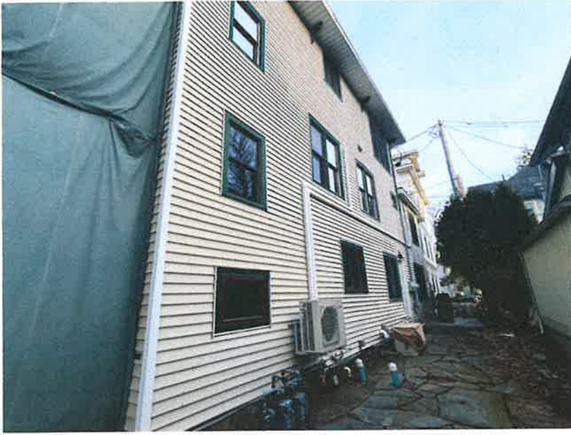
West side of building
